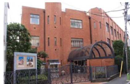
Main entrance Photo by Shoei
